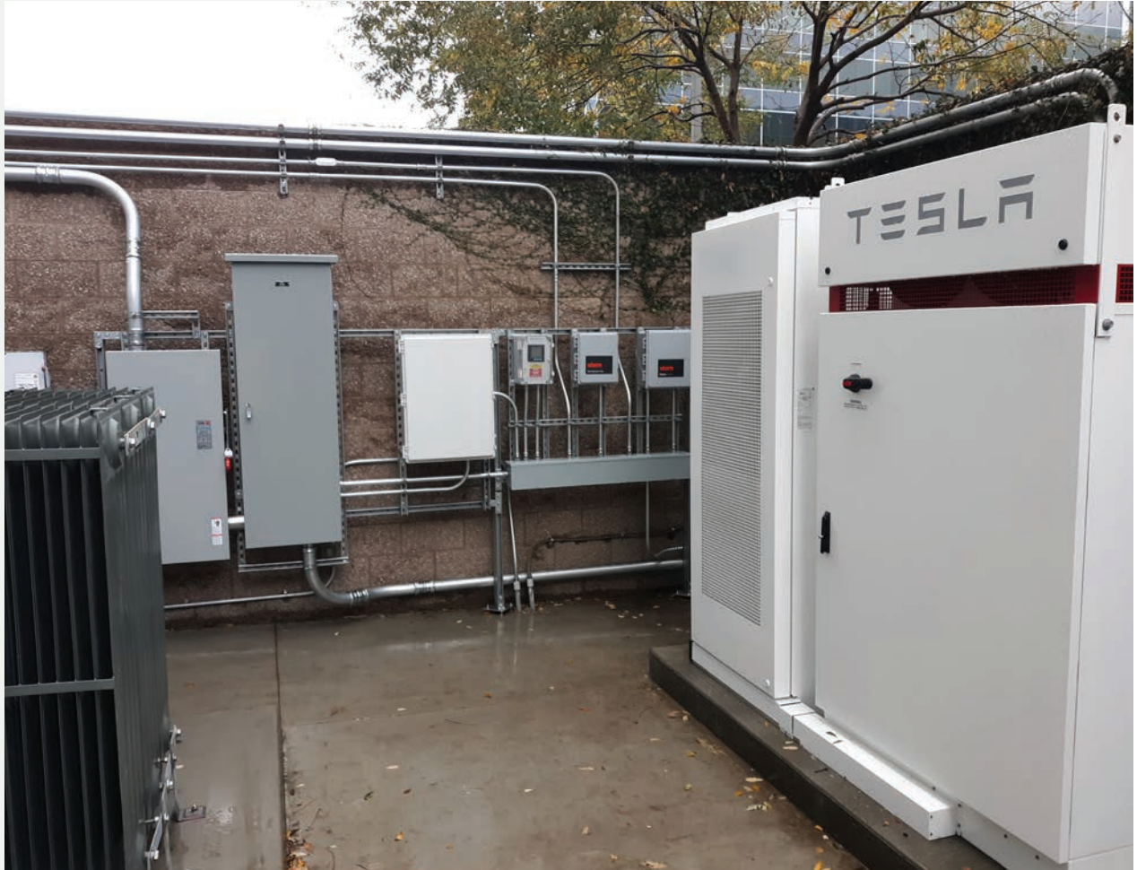
Tesla battery storage units at America Center.
